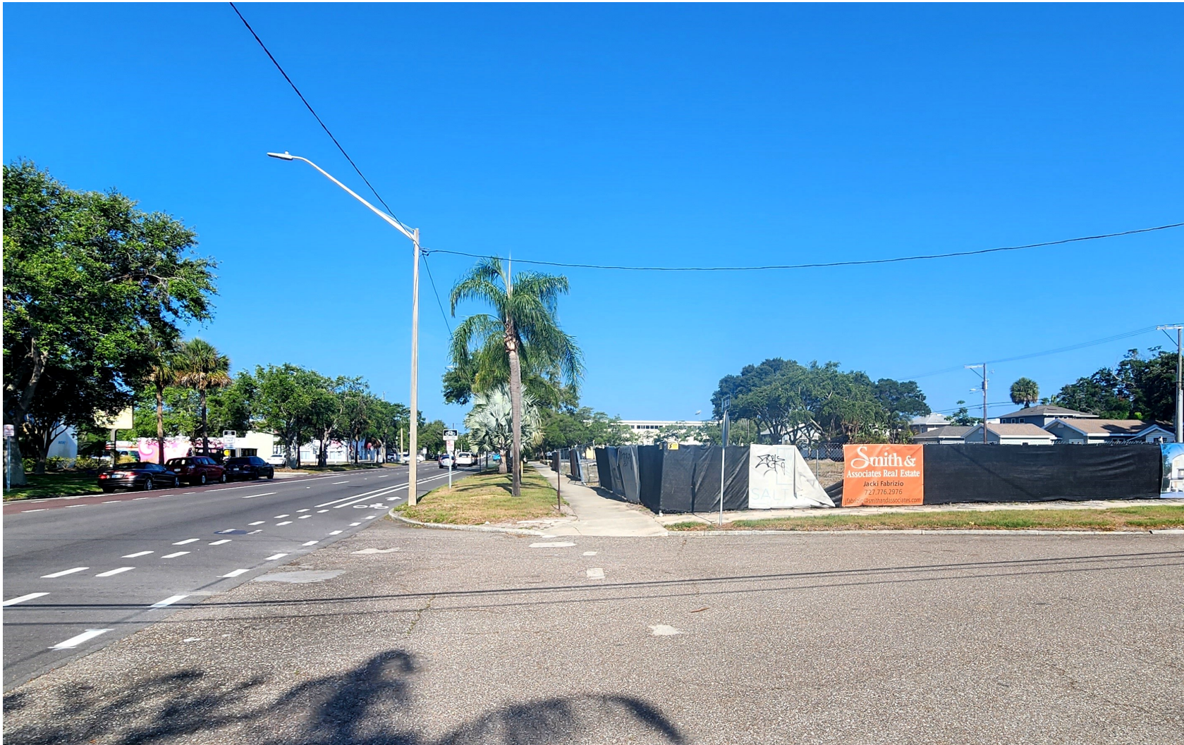
View of the corner looking westward
